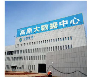
China Mobile data center
