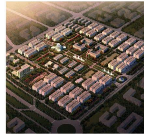
China Telecom data center
